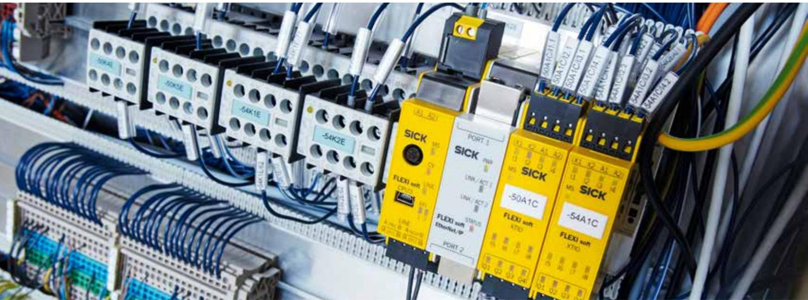
For nearly a decade Flexi Soft has been one of the best-selling safety controllers in industrial safety. It is freely programmable, easy to use, and can be expanded in a variety of ways with modular additions making it flexible and convenient. Compact and equipped with a network connection, Flexi Soft is the optimal solution for many machines.
