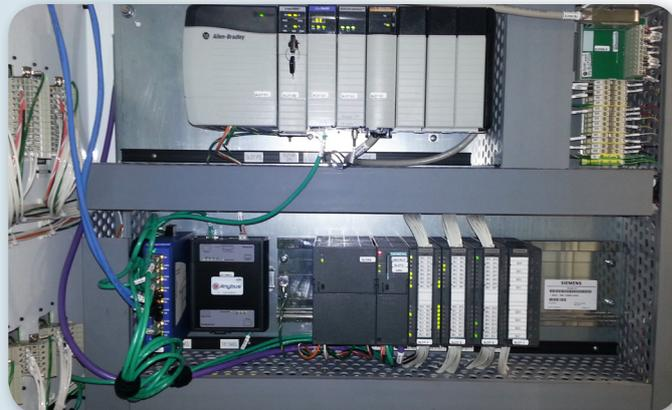
*The Anybus X-gateway allows Nagel's Allen Bradley PLC to communicate with any other industrial network. The above example uses a Slave-Adapter X-gateway between the EtherNet/IP-based equipment on the top rack and the PROFINET-based equipment on the bottom rack.*
